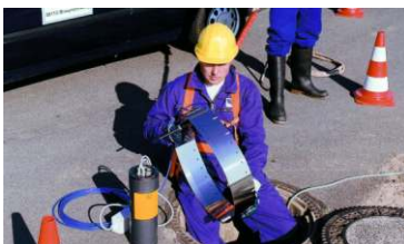
Installation of flowmeter
