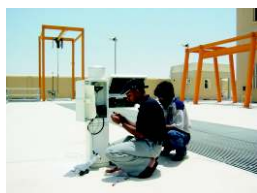
Installation of Telemetric Rain Gauge Station in Qatar
